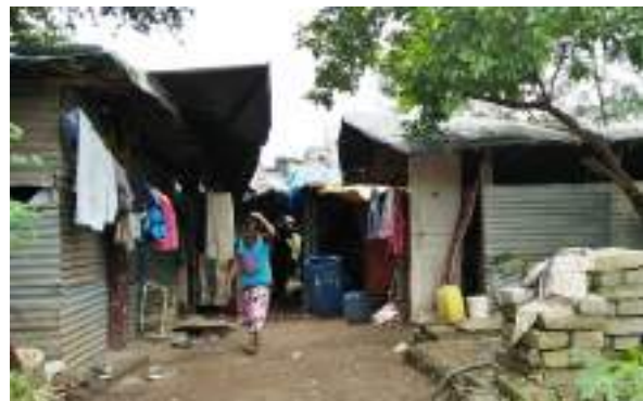
Picture 3.8 | Housing structures in Baltubai Nagar
