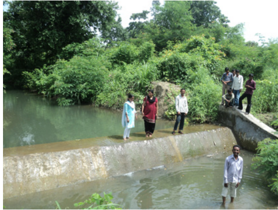
Cement nala bund constructed at Sarkinhi
